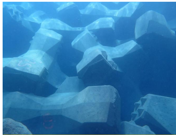
ACCROPODE™ II after installation
