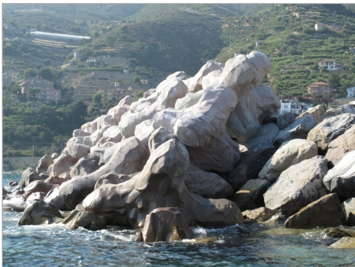
Above water ECOPODE™ armour in progress
