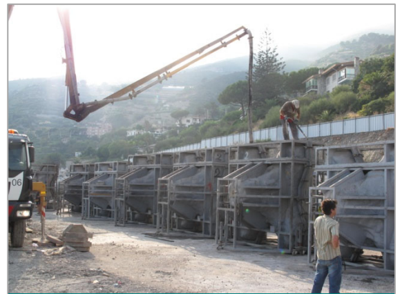
Casting of ECOPODE™ units
