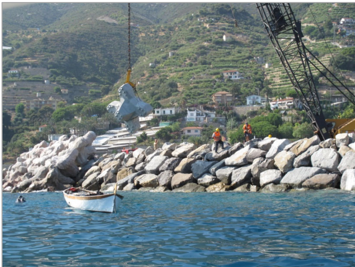
Placing of an ACCROPODE™ II unit underwater below ECOPODE™ units
