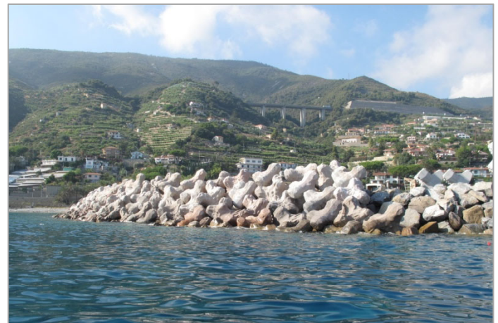
6 m 3 ECOPODE™ units placement in progress
