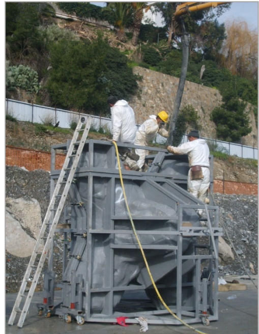
Casting using a chute
