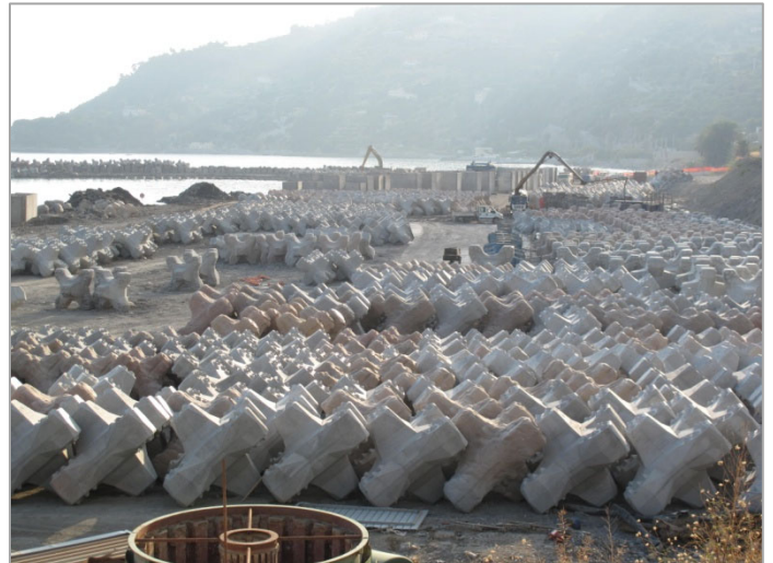
General view of the casting yard
