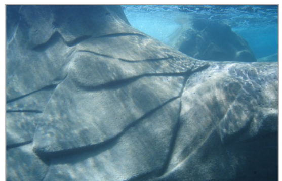
ECOPODE™ unit at the water level
