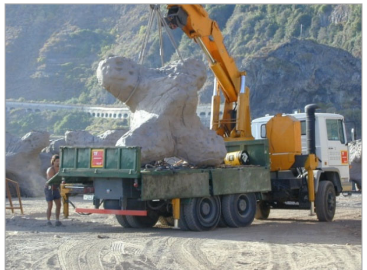
Transporting a unit on site
