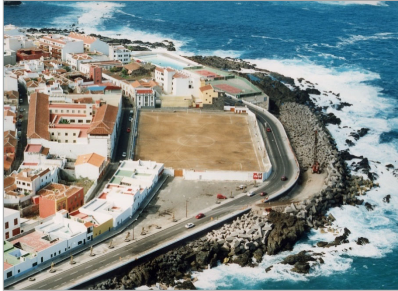
Placing of ECOPODE™ units at Garachico, Spain
