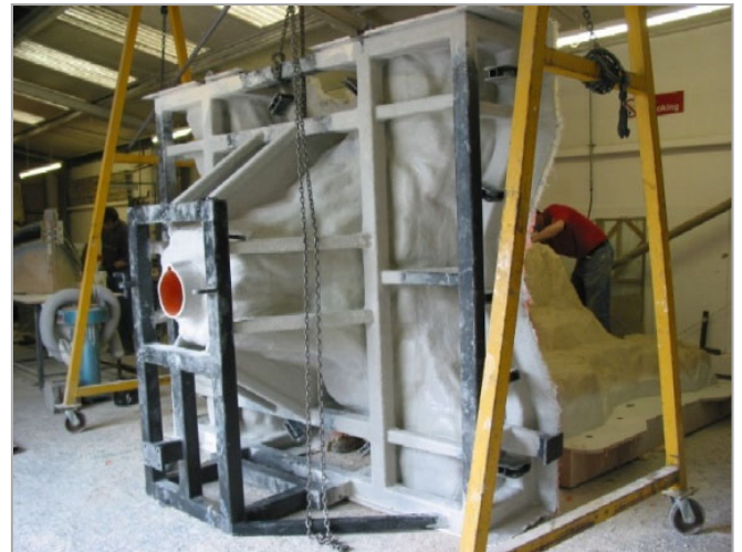
Assembling steel and fiber shells
