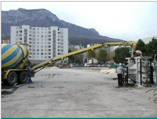
Casting with a conveyor belt
