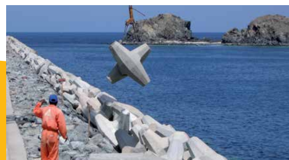
CORE-LOC™ armouring in progress
