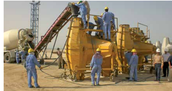
Casting using a conveyor belt
