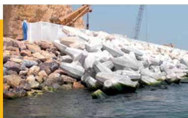
Placement in progress
