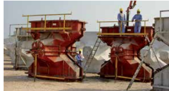
Form ready for casting
