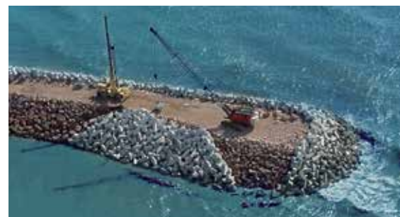
Placement in progress
